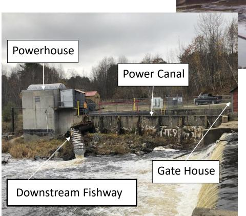
Rock Filled Timber Crib Dam
